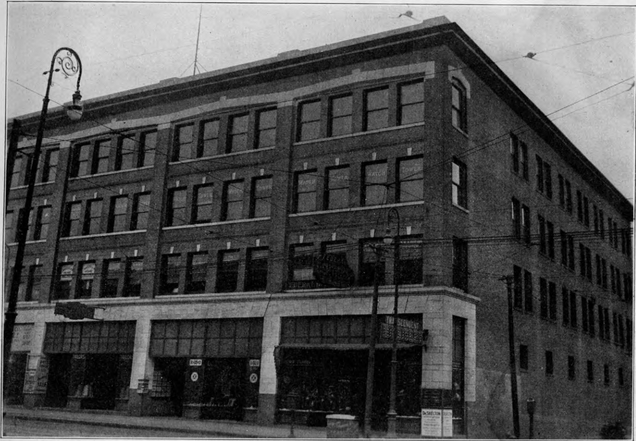
WATCH TOWER OFFICE
